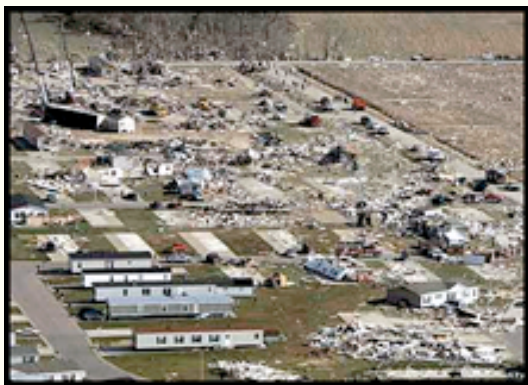
Evansville, Mobile Home Park hit by tornado, November 2005.
