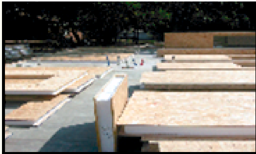
The house arriving on site.
